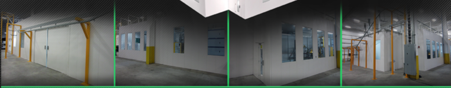
E-Room shown with automated conveyor system
